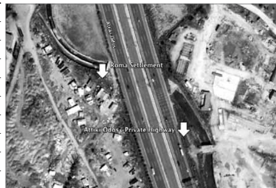
Terrain vague depicting the Roma settlement next to the private highway. Athens. 2010.
